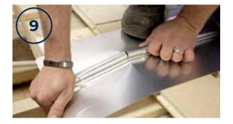
Use the folding points to cut the plates to the correct measure. Straighten any bent corners of the plates before installation.
