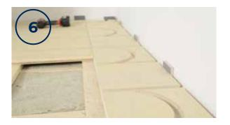
To allow for the wood's natural movement in service, the boards should be laid so, that a gap of at least 10mm is left between the boards and the walls and between the rooms. If the KoskiTherm boards are installed directly on battening, the extension joint of a turn board should be installed and screwed on the battening. When installing on spaced boarding, the extension joint of a turn plate should not necessarily be on top of the battening.
