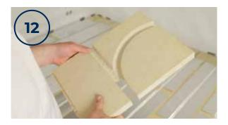
The inlets are milled before installation of the boards or directly to the floor surface.
