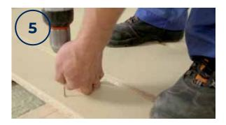
The KoskiTherm boards should be screwed to the base with screws suitable for screwing wood. The screws should be countersunk screws 50–75mm in length. The screws are attached to the middle and the edges of the boards 300–450mm apart.
