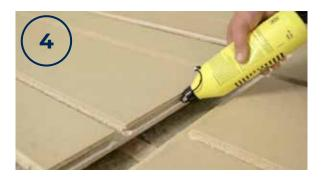
The boards should always be glued to each other at the tongue and the groove. The boards can also be glued to the base to avoid possible creaking. The glue should be an appropriate PVA wood glue. Application of the glue should be done carefully ensuring that there is a continuous seam of adhesive along the entire length of the tongue and groove. Note however that excessive use of glue might lead to gaps between the boards.
