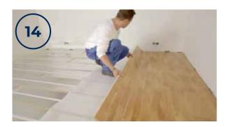
Both parquet and laminate can be installed directly on the heat transfer plates and footfall sound insulation. In the case of other surface material solutions, construction boards of at least 6mm in thickness should be used.
