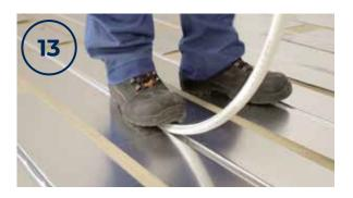
Install the heating pipes into the grooves of the heat transfer plates. Make sure, that the pipe is fully embedded to the groove to avoid it carrying load under the final floor surface.
