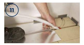
The installation of the heating pipe is begun by passing it through the floor to the manifold.
