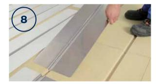
The heat transfer plates are installed by pressing them to the straight sections of KoskiTherm boards. The distance between the heat transfer plates has to be 10–100mm. There is no need to attach the heat transfer plates to the base.
