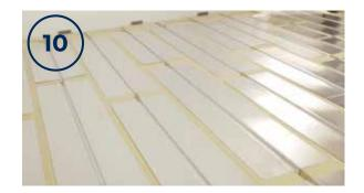
70-90% of the floor area should be covered by the heat transfer plates. The floor should be cleaned once more before the installation of the pipework.
